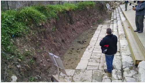
Partially excavated Pool of Siloam today
